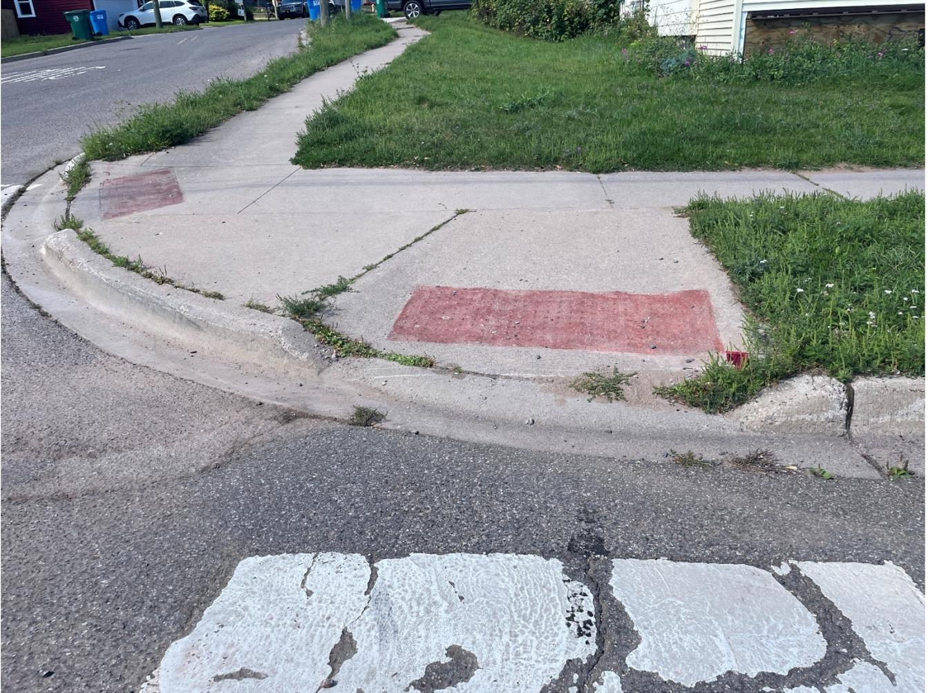
**Image 19: Curb ramps at an intersection corner**
