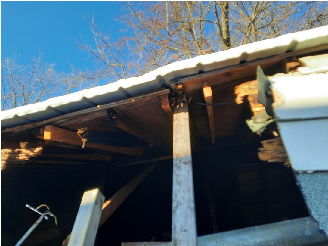
2 - Unsupported roof framing
