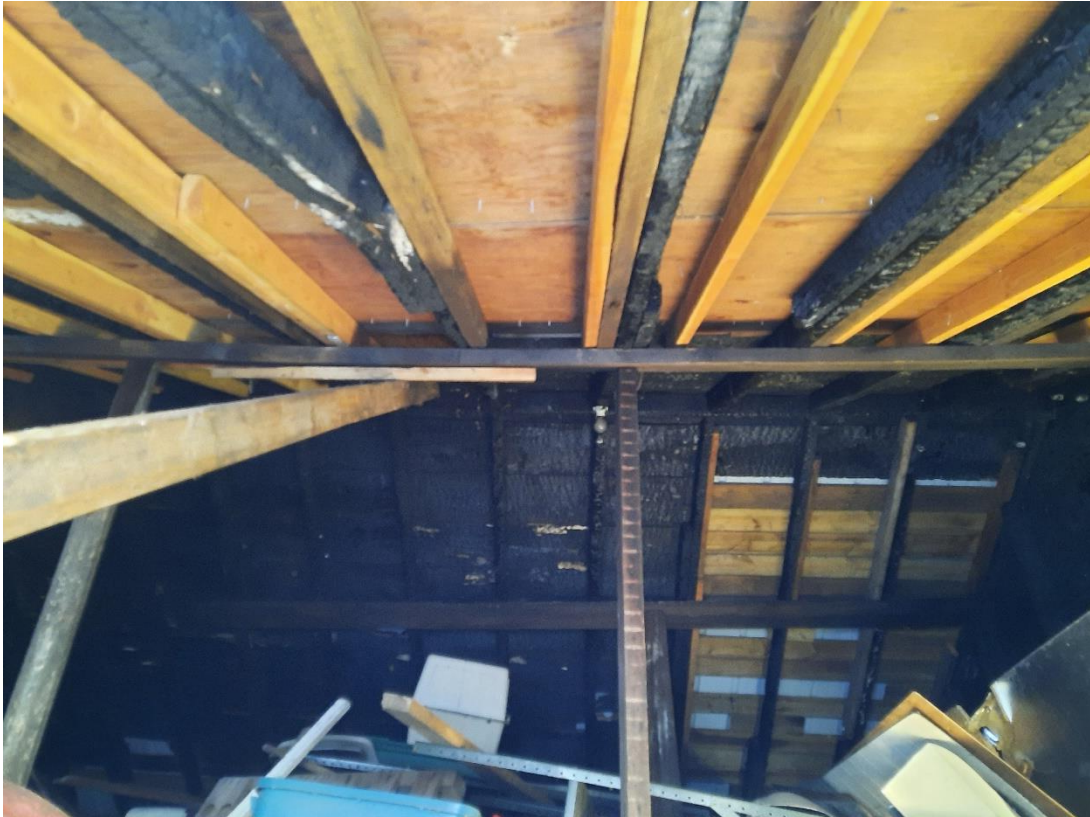
3 - Charred roof framing
