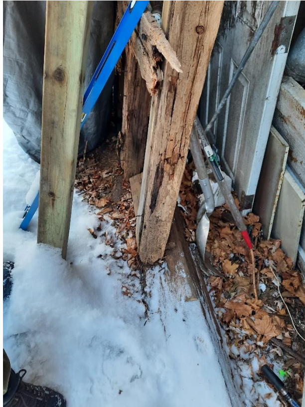
5 - Sill rotated out of position
