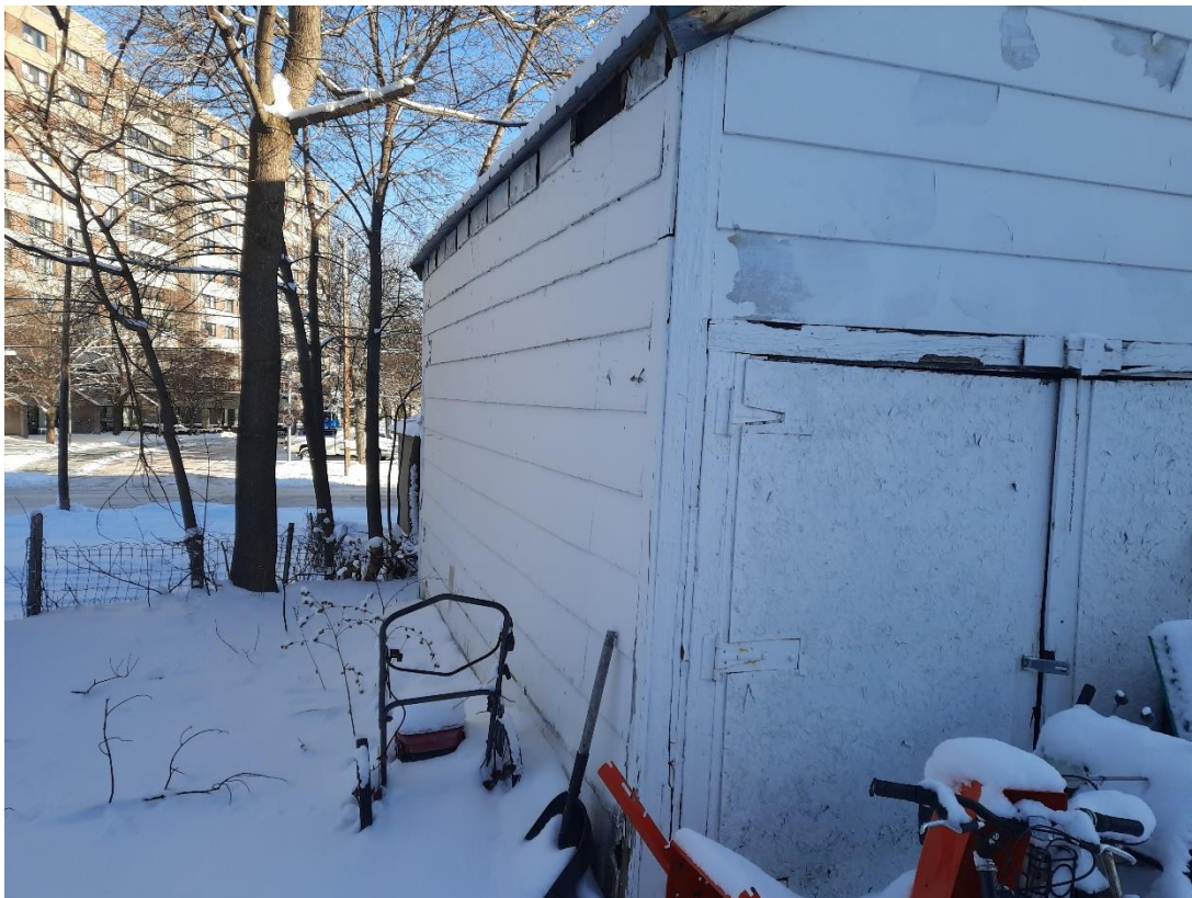
6 - West wall bowing out due to collar tie failure
