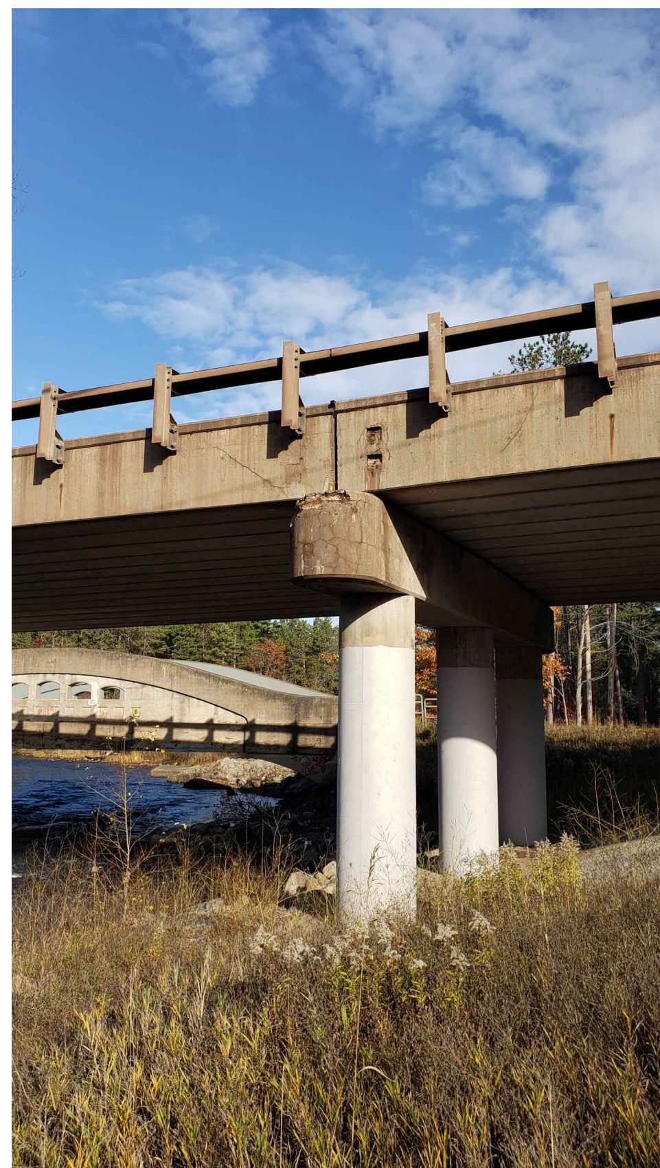
SOUTHEAST PIER CAP
