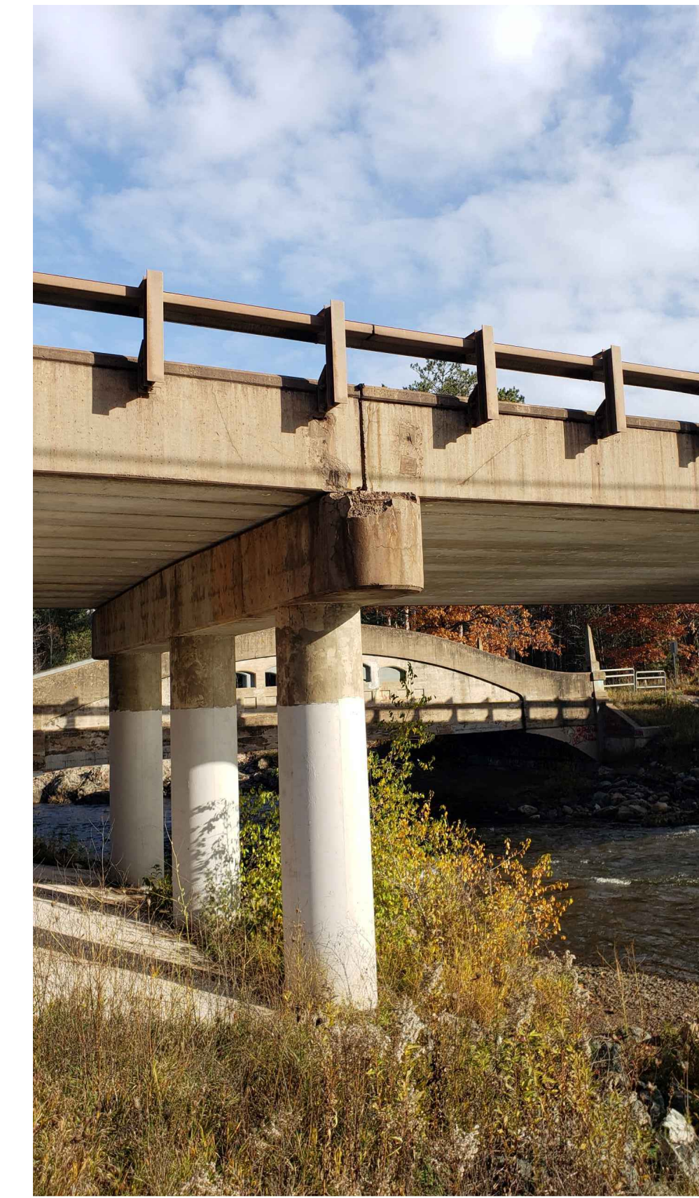
SOUTHWEST PIER CAP
