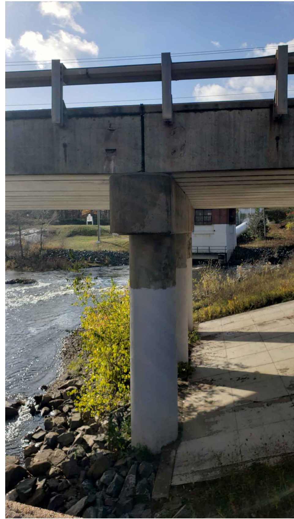
NORTHWEST PIER CAP
