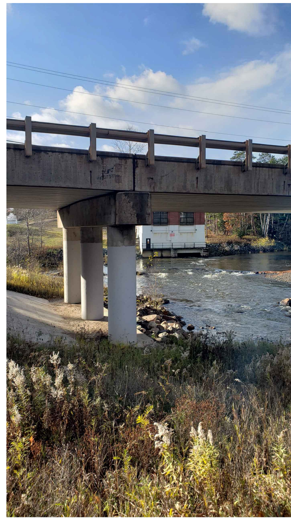
NORTHEAST PIER CAP
