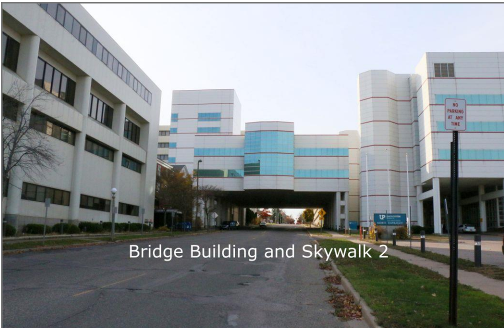
Figure 5. Bridge Building, view to the west
