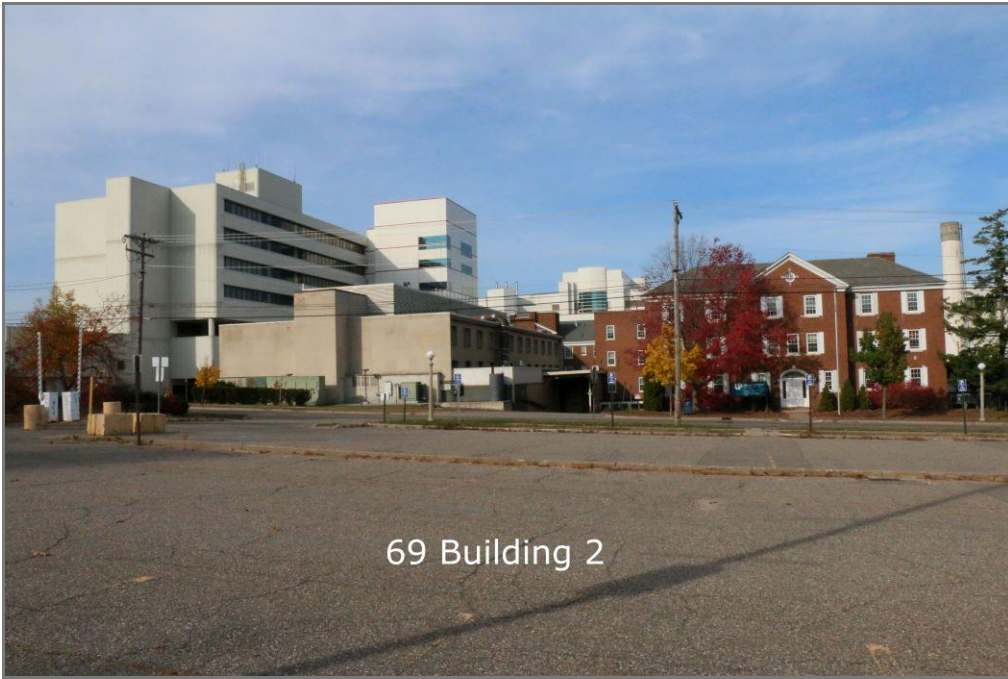
Figure 9. South Tower (81 Building), Patient Care Building (69 Building), and Wallace Building, view to the northwest
