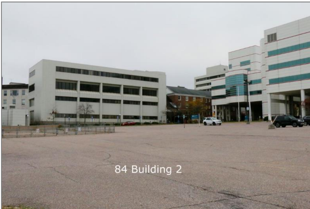
Figure 5. East Building (84 Building), view to the southwest
