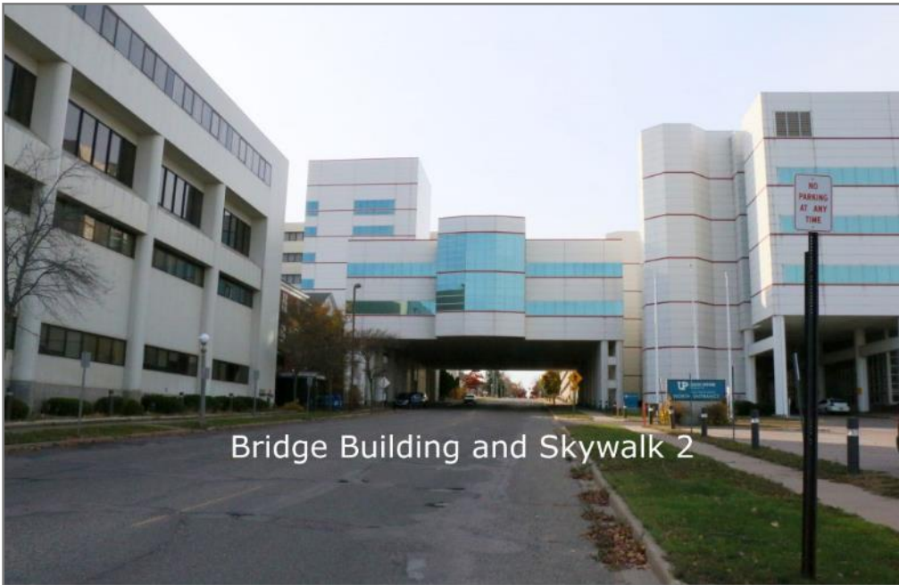
Figure 7. Bridge Building, view to the west
