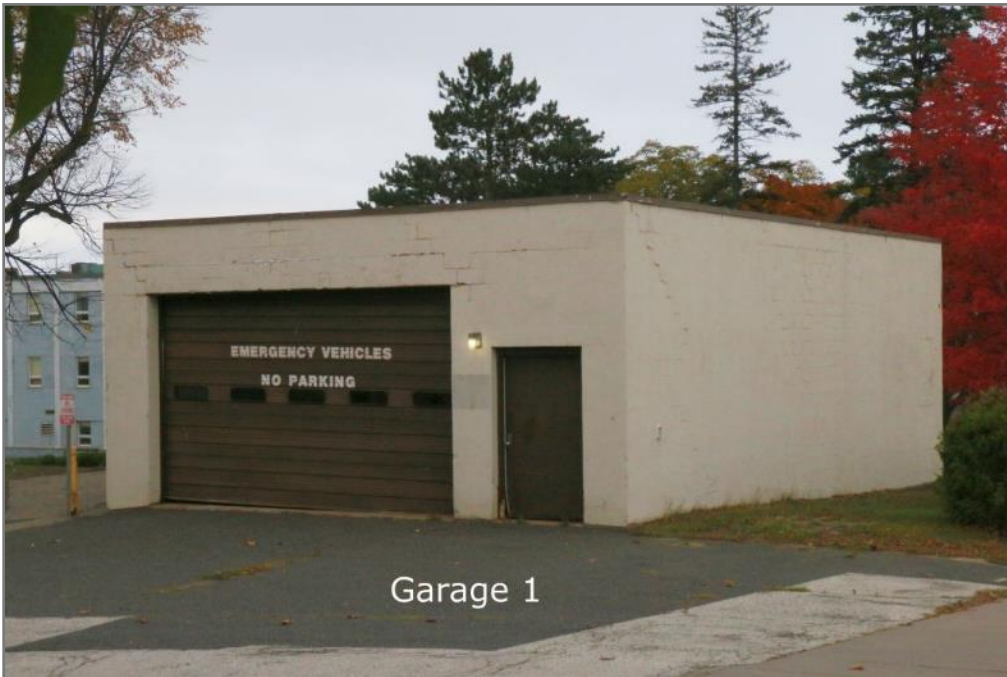
Figure 15. Garage, view to the northeast
