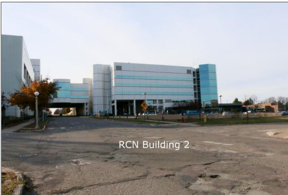
Figure 8. Bridge Building and Robert C. Neldberg Building (RCN Building), view to the northwest
