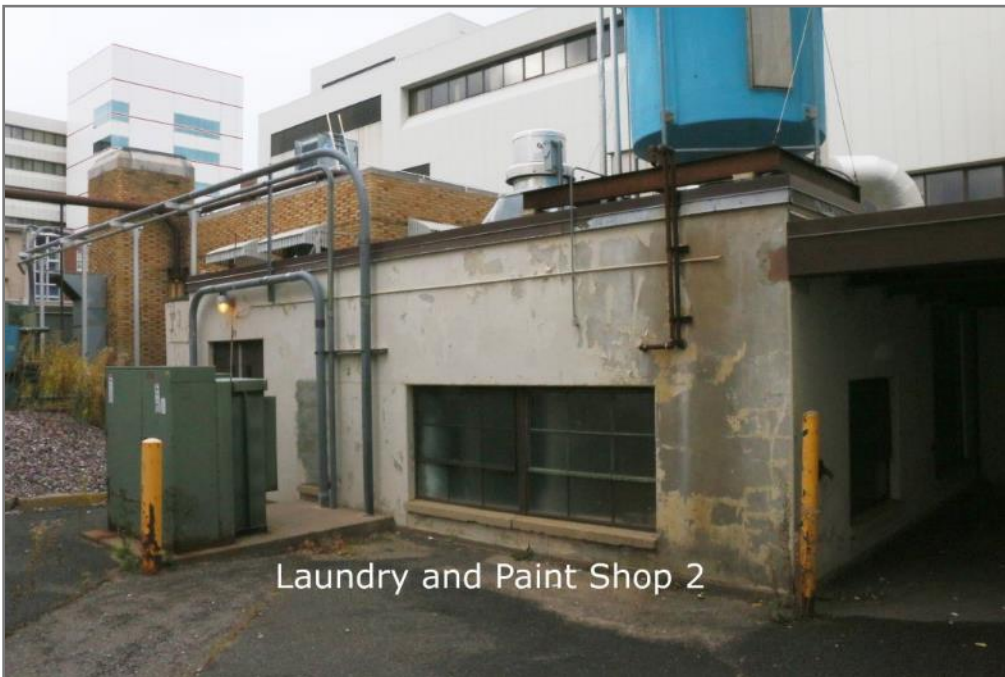
Figure 14. Paint Shop and Laundry, view to the northwest
