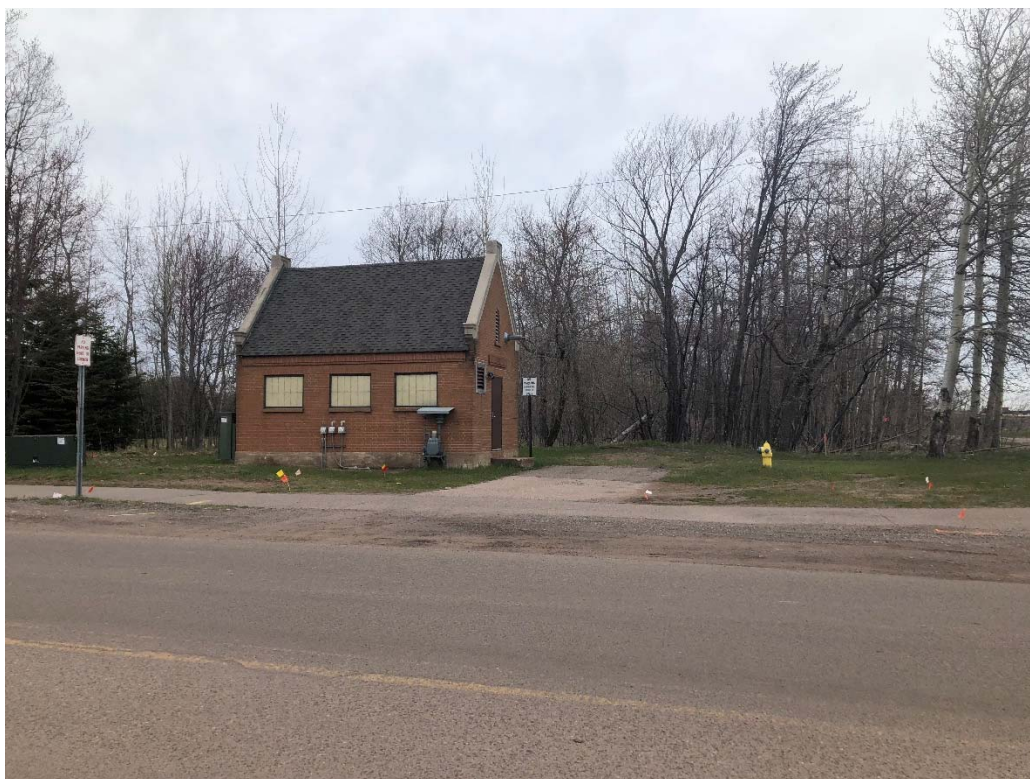
Photo 8. Looking north at the City municipal pump house building located near the northwest intersection of Hawley Street and Lakeshore Boulevard (date of construction is unknown).
