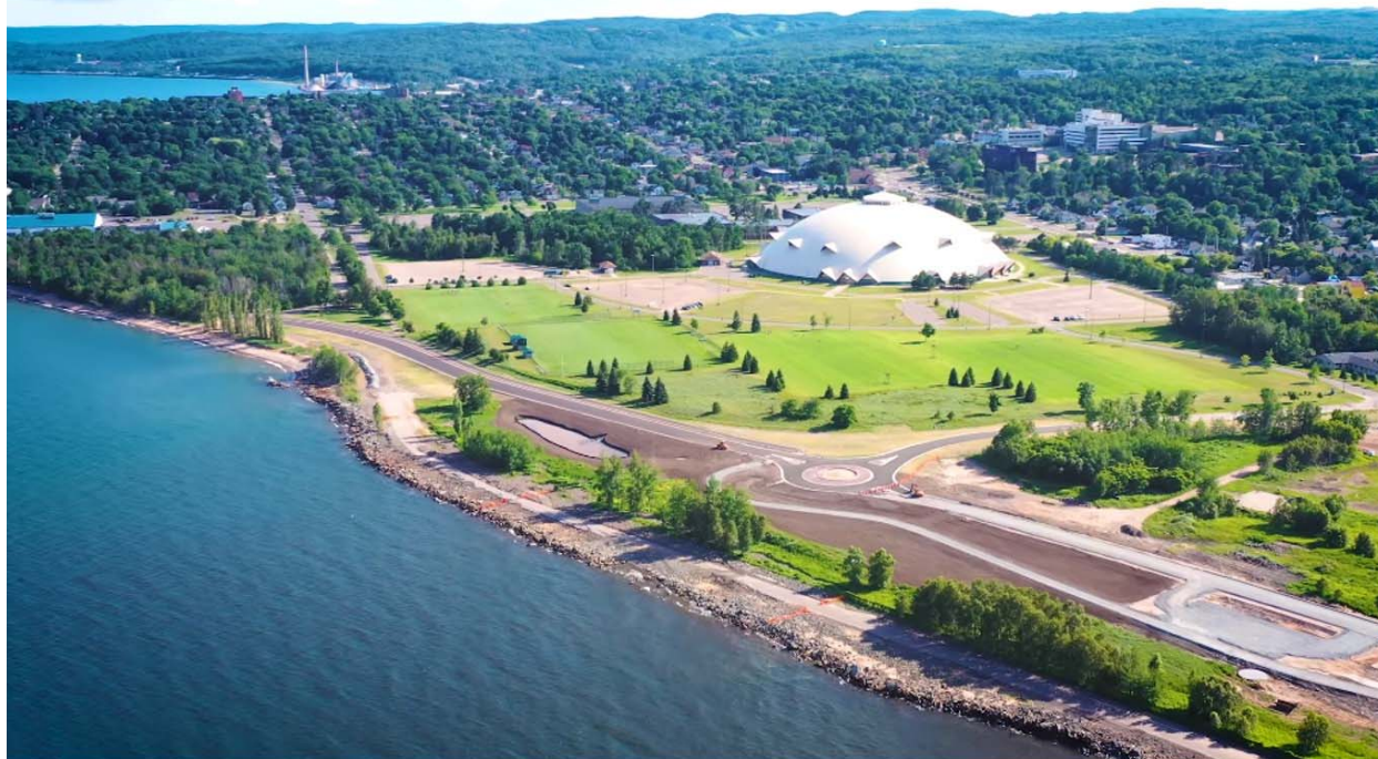
Photo 21. Aerial photo looking southwest at the coastal restoration/beneficial reuse area (July 2020). Phase I included road relocation to move the road inland. Phase II shoreline restoration to begin in 2022.
