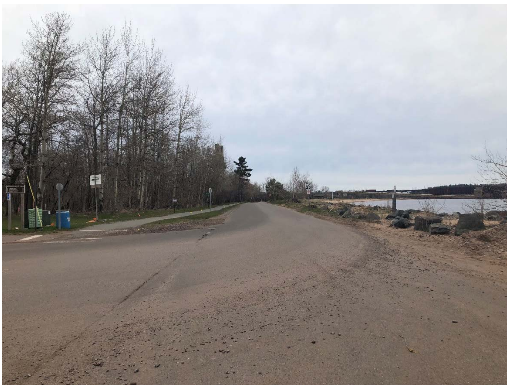
Photo 9. Looking north at the Port access road (Lakeshore Boulevard) at the intersection with Hawley Street.
