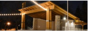
The Cedar Creek Park Band Shell re-places an existing 50-year old band shell in an effort to improve Cedar Creek Park. The new stage features a cantilevered slab that is supported in part by the existing band shell founda-tions as-well-as the new multi-glulam column moment frame featured at the front of the stage. The exposed glulam roof joist and beam structure combines architectural aesthetics with structural purpose.
